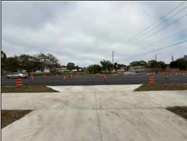
View of E University Blvd
