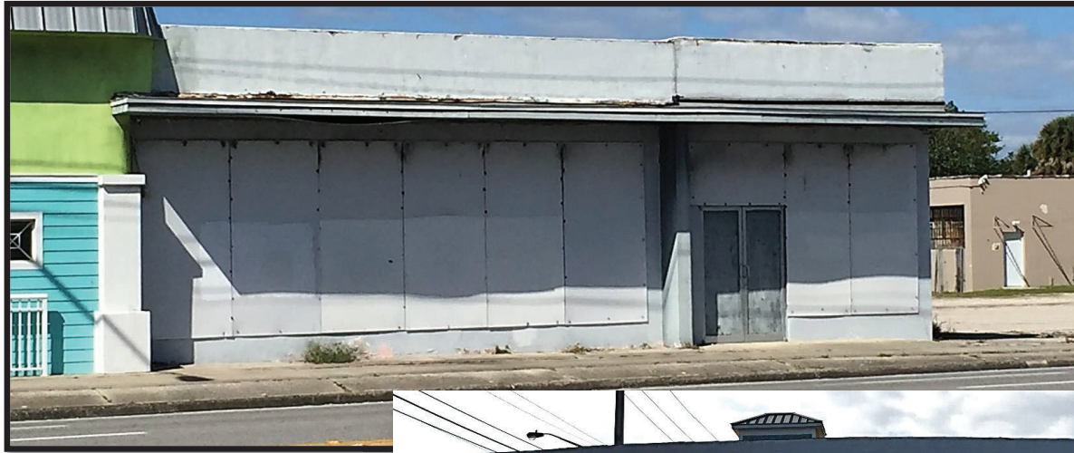
Existing Front, East Façade - US 1/Harbor City Blvd.
